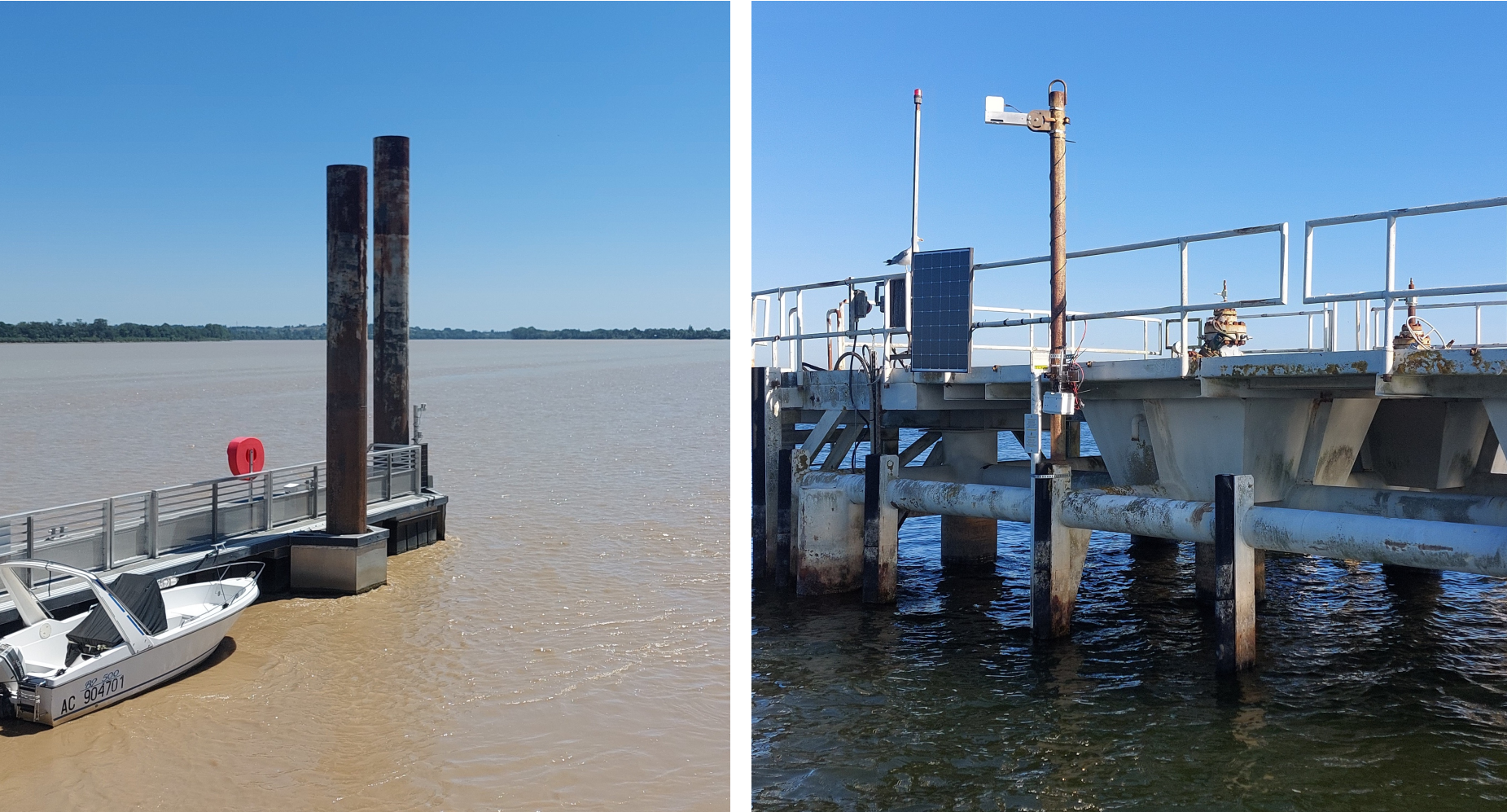
Platforms at Dordogne River (left) and Parentis Lake (right), France
