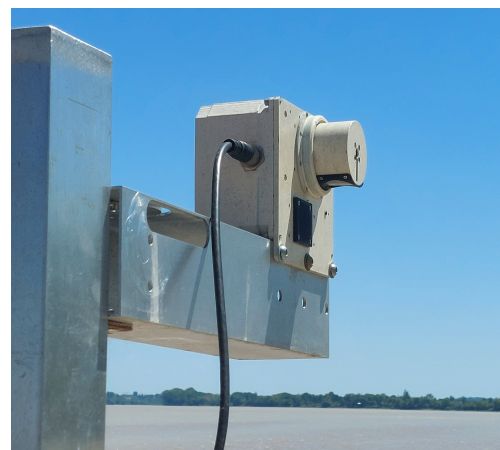
MHR.2 INSTALLED ABOVE THE WATER
